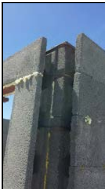
Photo 7.9 Interior Corner, 10" Asymmetric ICCF
