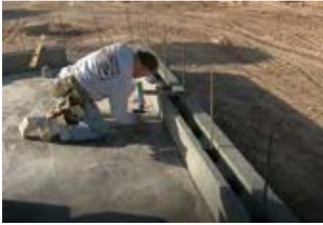
Photo 7.6a Tack gluing (every 12") of the first course.
