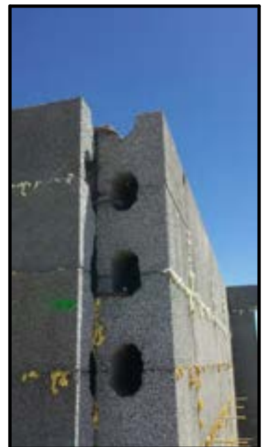
Photo 7.10 Exterior Corner, 10" Asymmetric ICCF
