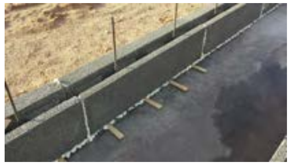
Photo 7.6c Plumb and level and polyurethane foam adhesive in place. Take great care not to move the block when tacking block in place. 15 to 20 minutes later, when the tack gluing dries, you can "super glue" (glue every 3-4") the block.
