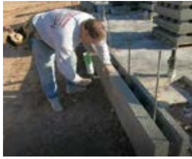
Photo 7.6b Tack gluing, both sides.
