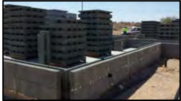
Photo 7.8 The second course placed, plumbed, leveled, and glued. (10" Asymmetric Block pictured)
