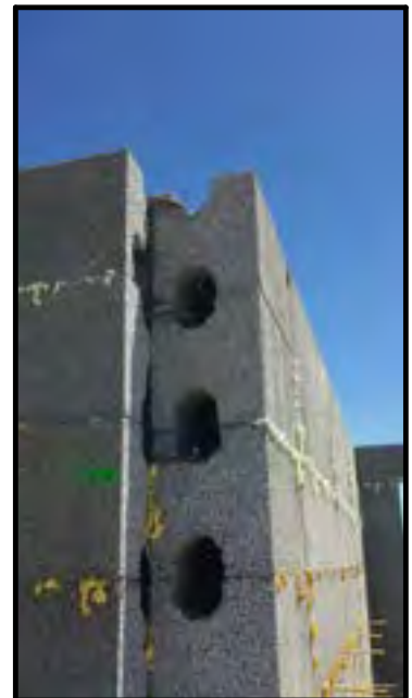
Photo 7.10 Exterior Corner, 10" Asymmetric ICCF
