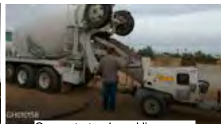
Concrete truck and line pump
