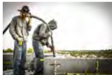
Concrete truck and line pump
