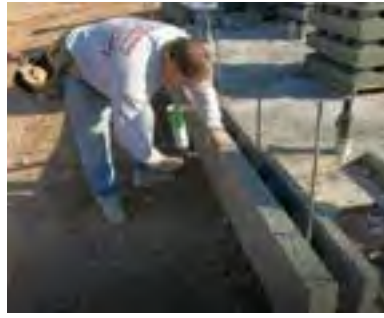
Photo 7.6b Tack gluing, both sides.
