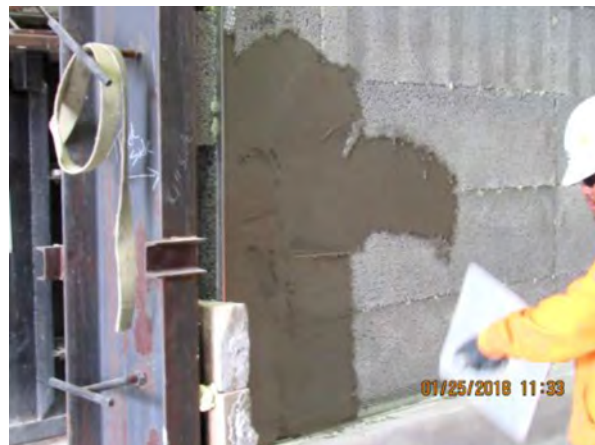
Brown coat being keyed into bare ICCF block, 5/8" to 3/4" thick.
