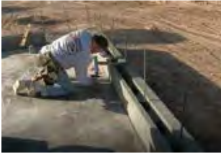
Photo 7.6a Tack gluing (every 12") of the first course.
