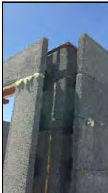
Photo 7.9 Interior Corner, 10" Asymmetric ICCF
