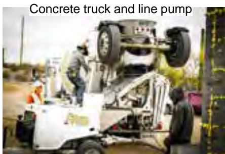
Concrete truck and line pump
